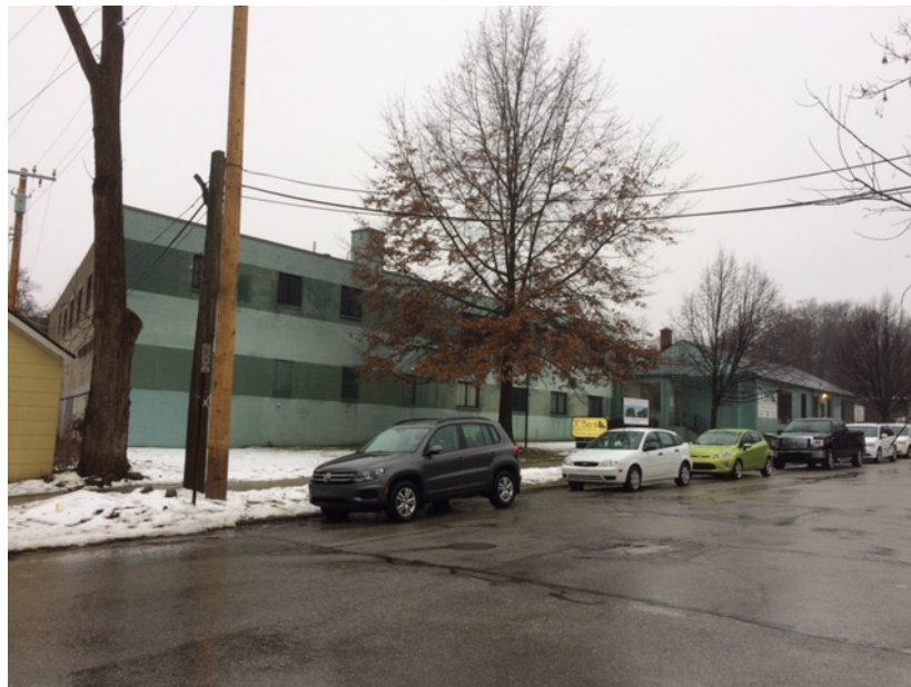
CURRENT SITE from Felch side
