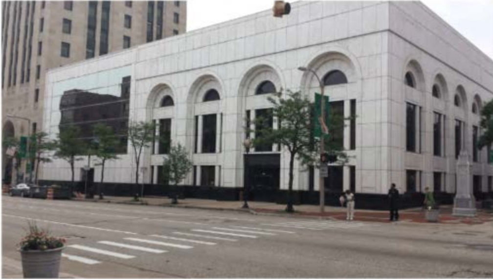
Front of Building facing E. Michigan Avenue
